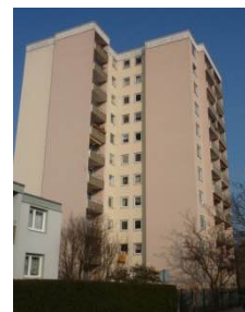
Figure 2. Building with a cable-driven elevator
